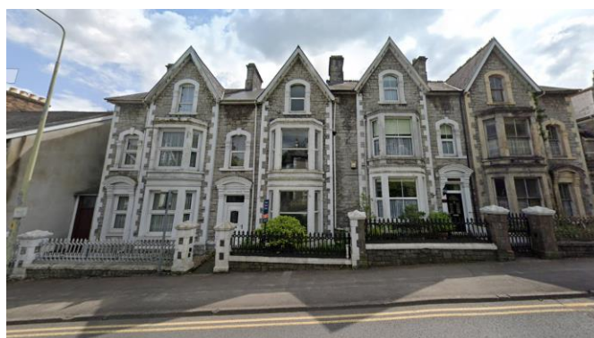
Fig. 2: Photo showing Front elevation of 61 Park Street
